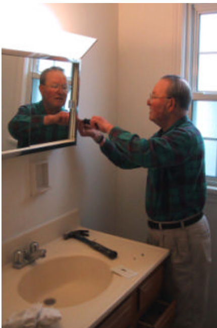
Lou helped out in the Jim Kubarek bathroom
